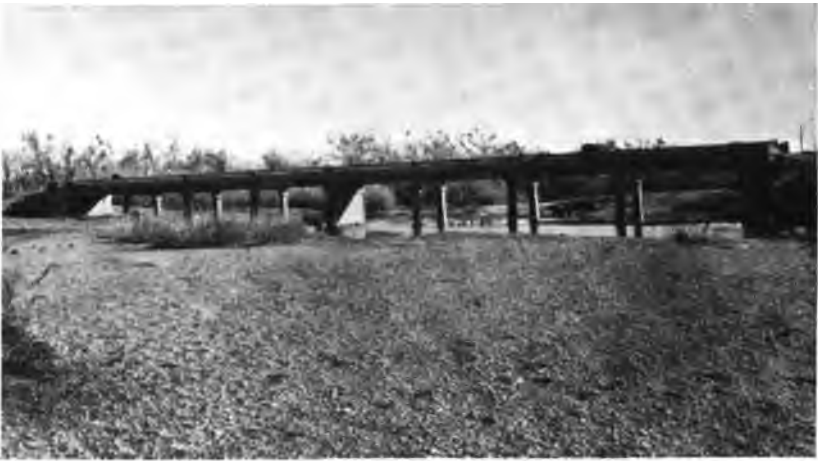
This structure and the one shown above were built by county forces and cost much less than the lowest contractor's bid.
